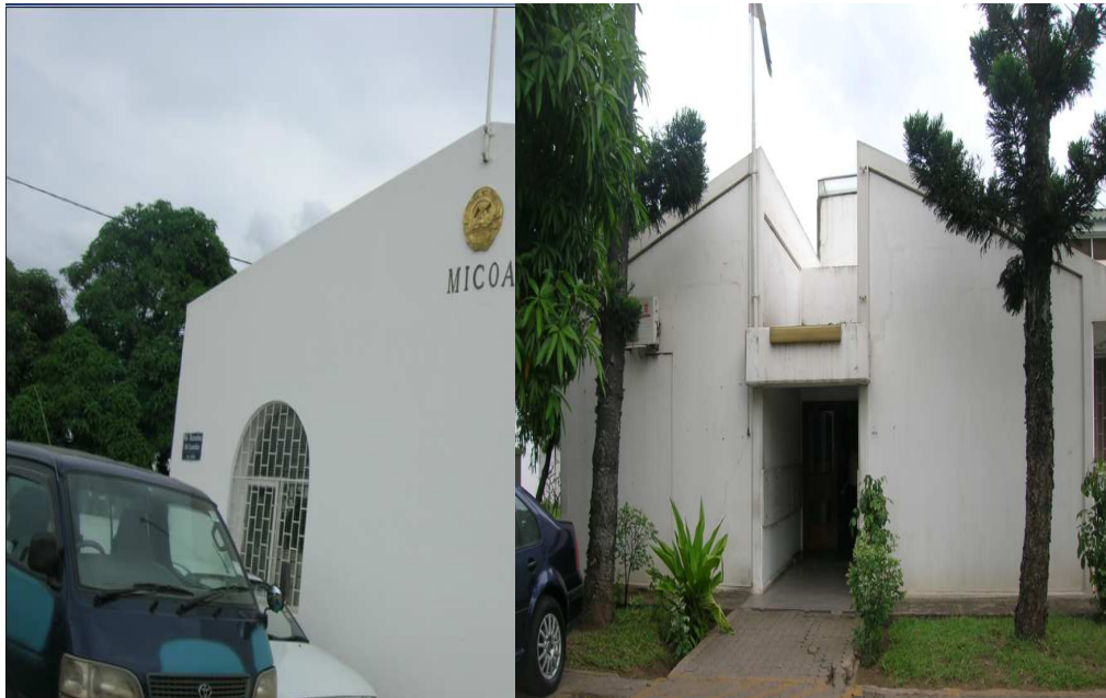
Figure 5 Installation of MICOA where the DINAPOT is
