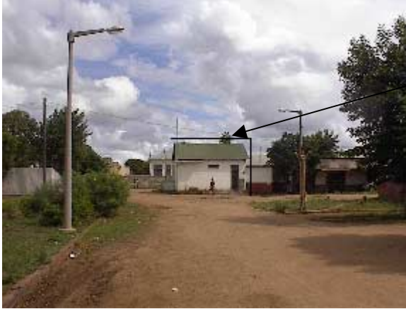
Picture 6.6 – District Warehouse in Moamba
