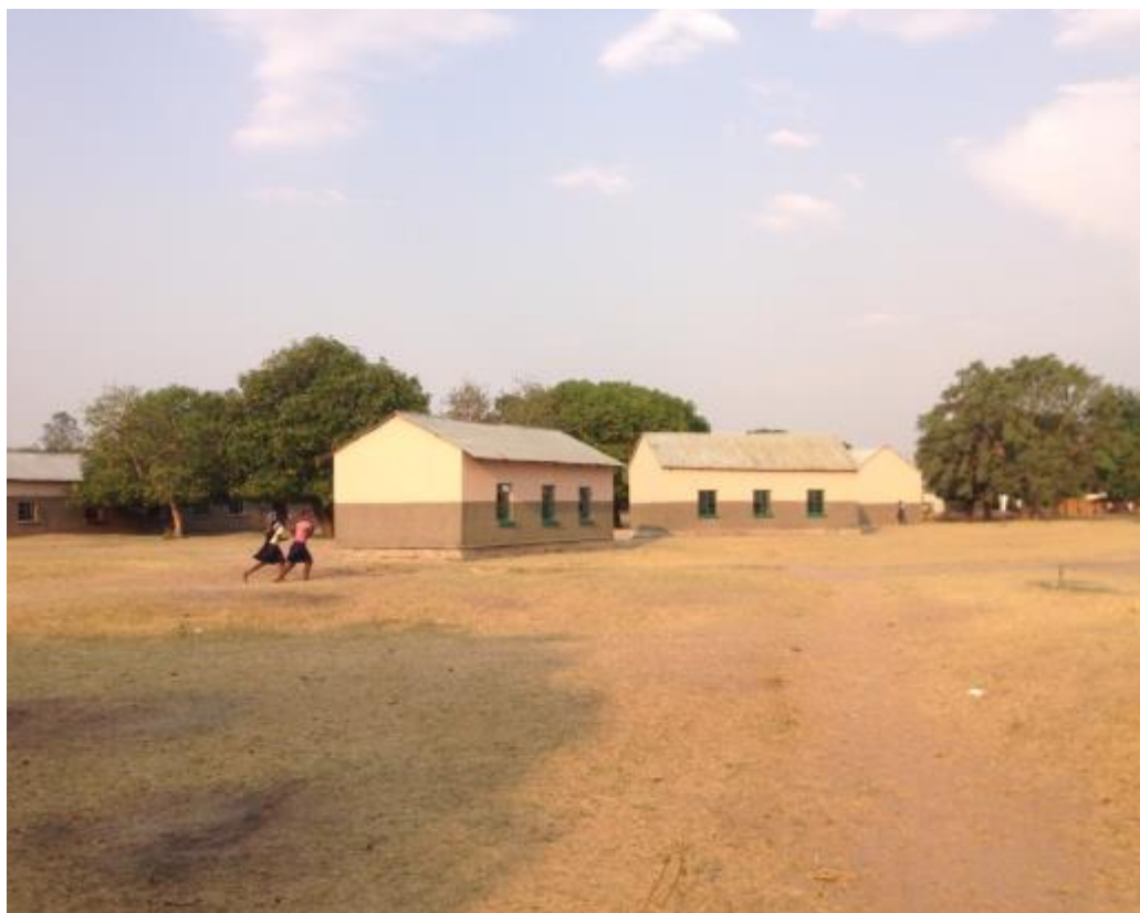
Figure 6.1 Public school in rural Zambia
